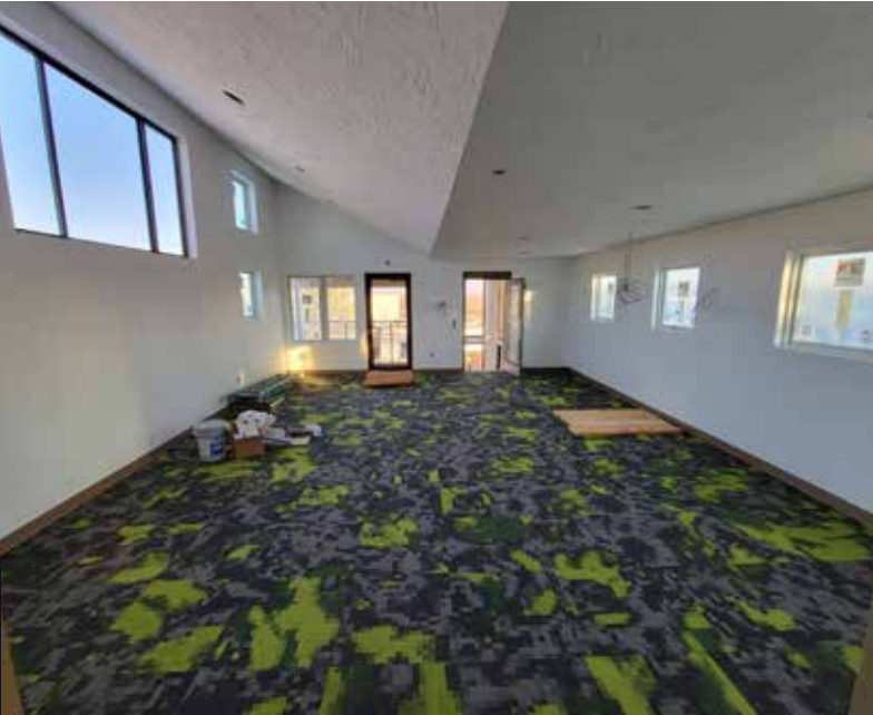
Newly completed interior
